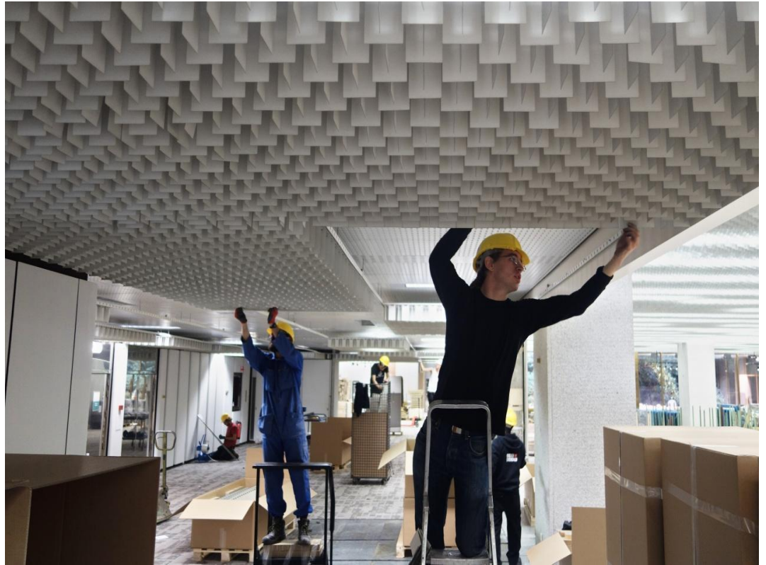
Fig. 5.7.1 Dismantling of interior fittings at the former headquarters of BNP Paribas Fortis Source: Rotor Deconstruction's website, 2014-2016.
