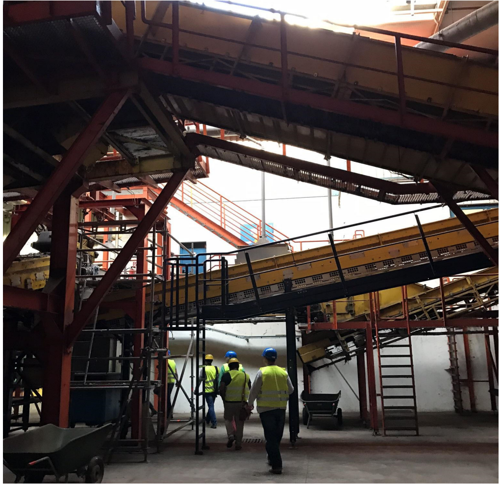
Figure 6.2 Biowaste treatment plant of GAB (HCU Team, 2018).
